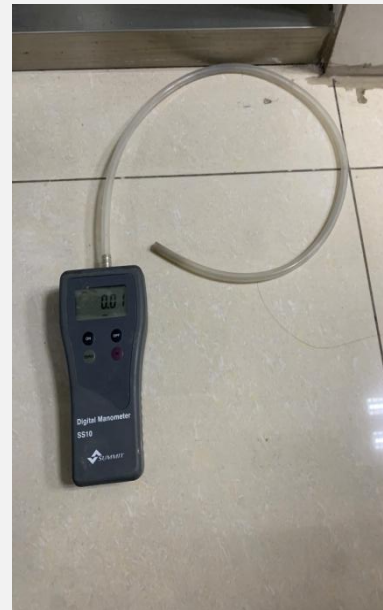
气压检测 Gas pressure test
